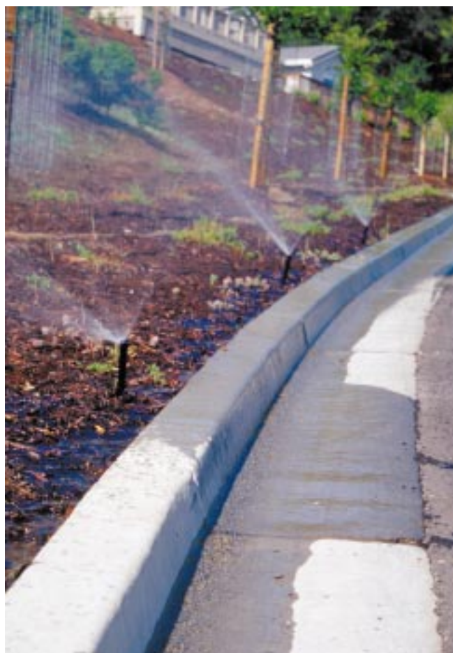
Not all water applied to landscapes is used by plants. Some is lost due to runoff, windspray, or deep percolation. Irrigation efficiency losses need to be included in water budget calculations.
