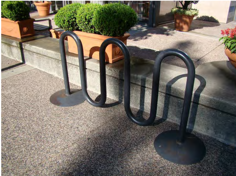
This bike rack is installed too close to the bench, not providing the recommended 36 inch horizontal clearance needed to accommodate most bikes.
