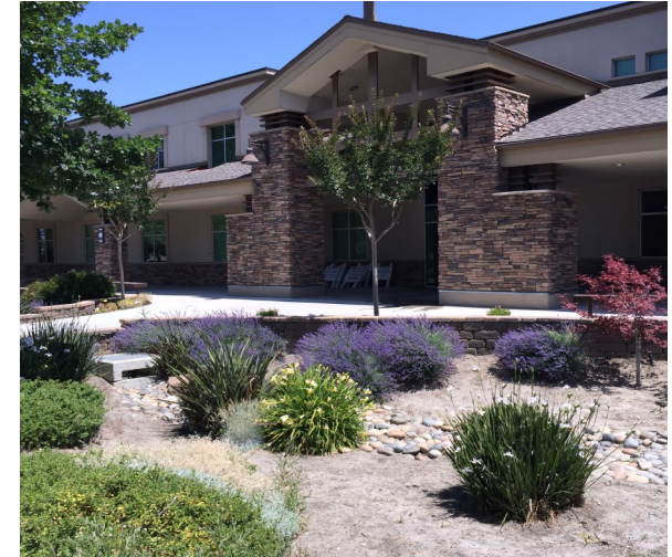
Stormwater Treatment, Bioretention Basin
