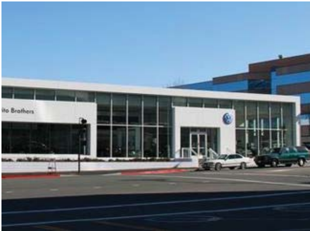
Auto showroom along sidewalk with transparent frontage and pedestrian entrances
