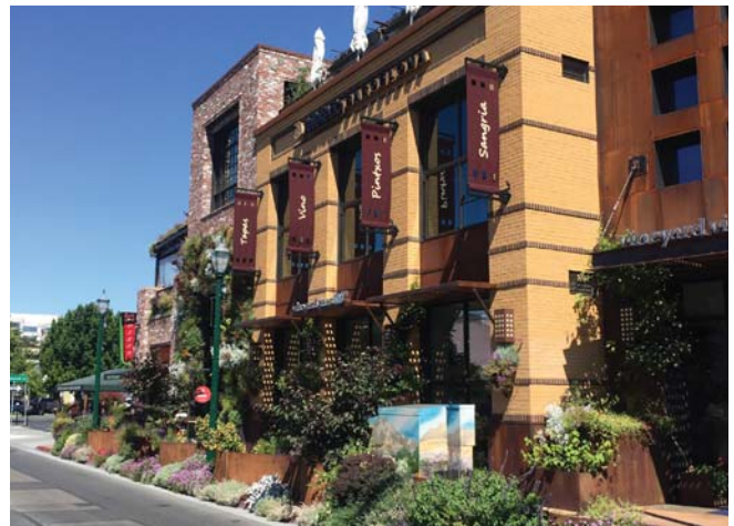
Vertical and horizontal articulation through use of structural bays and variation in roofline, setbacks, color, and materials
