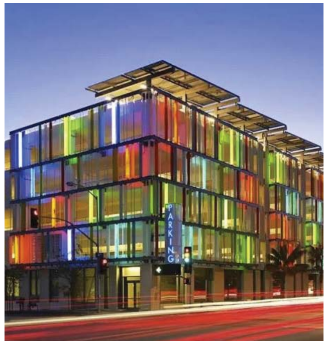
Unique parking structure design
