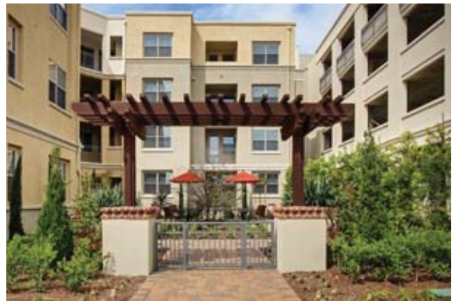
Example of entrance fencing along residential development
