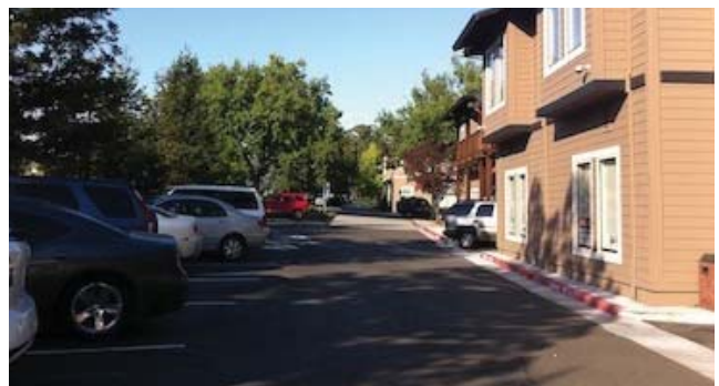
Parking lot located behind building
