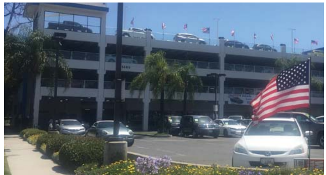
Shared parking structure for auto dealership inventory
