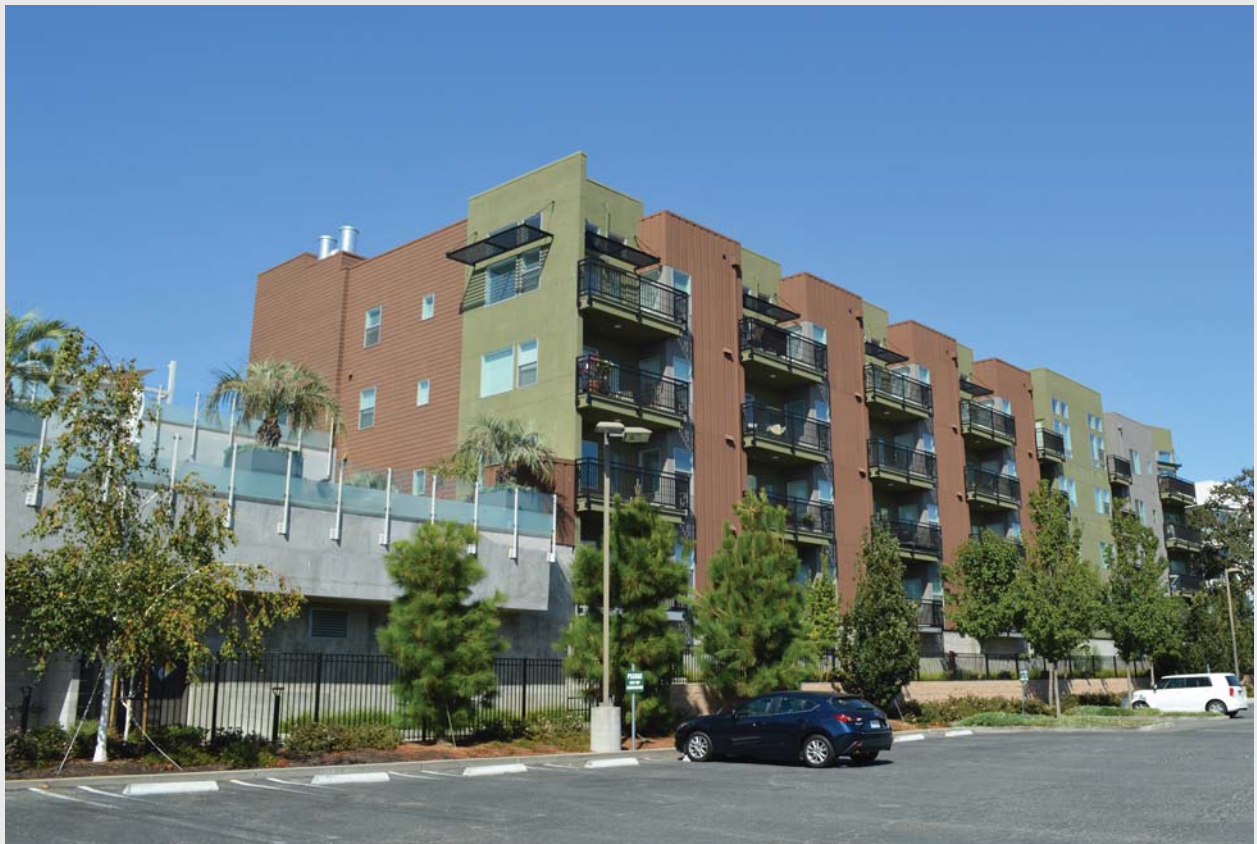
The Ave project (formerly “Ascent”) was built in accordance with different Measure A height maximums that applied to different parts of the same parcel
