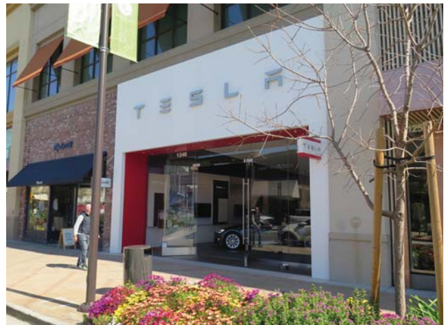
Well integrated retail frontage that incorporates auto sales
