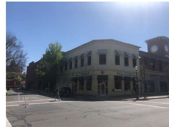
CORNER OF DUNCAN ST NORTH MAIN ST
