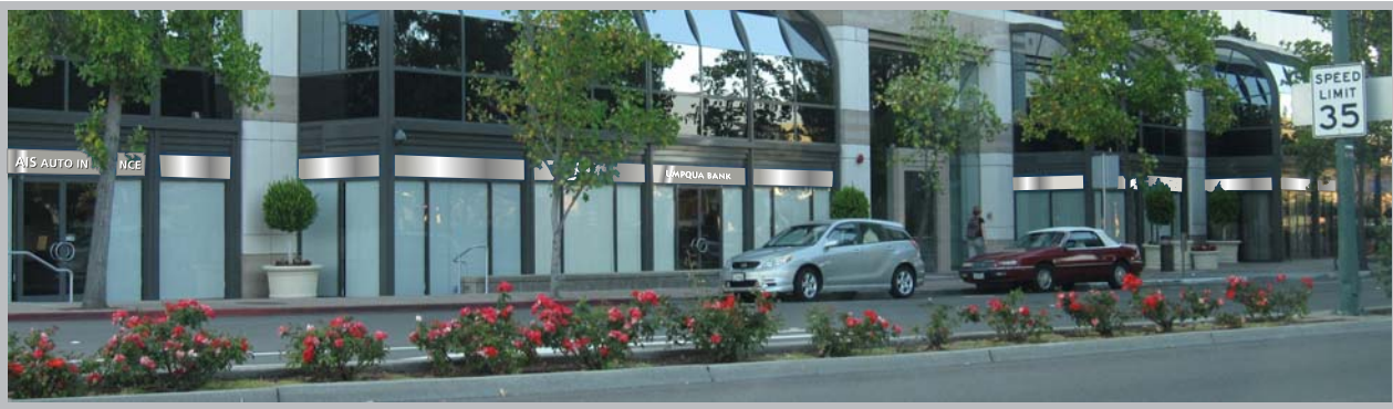
1333 N. CALIFORNIA VIEW | SOUTH END OF BUILDING
