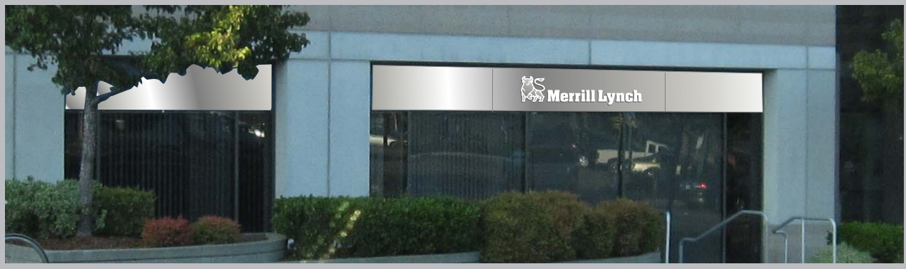
1331 | MT. DIABLO VIEW | WEST END OF BUILDING
