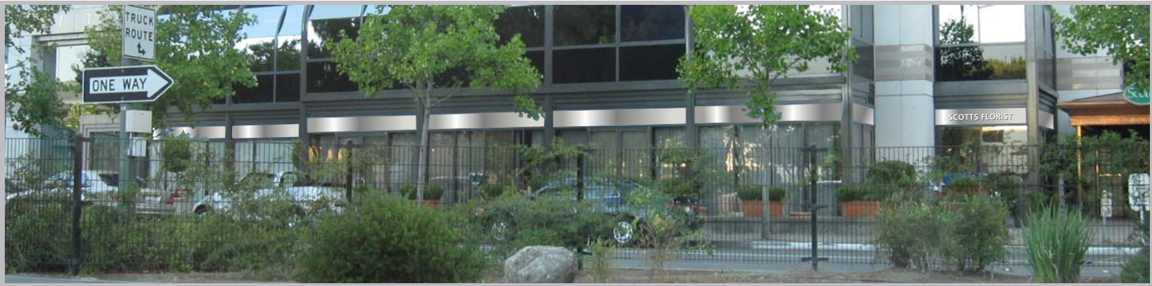
1333 N. CALIFORNIA VIEW | NORTH END OF BUILDING
