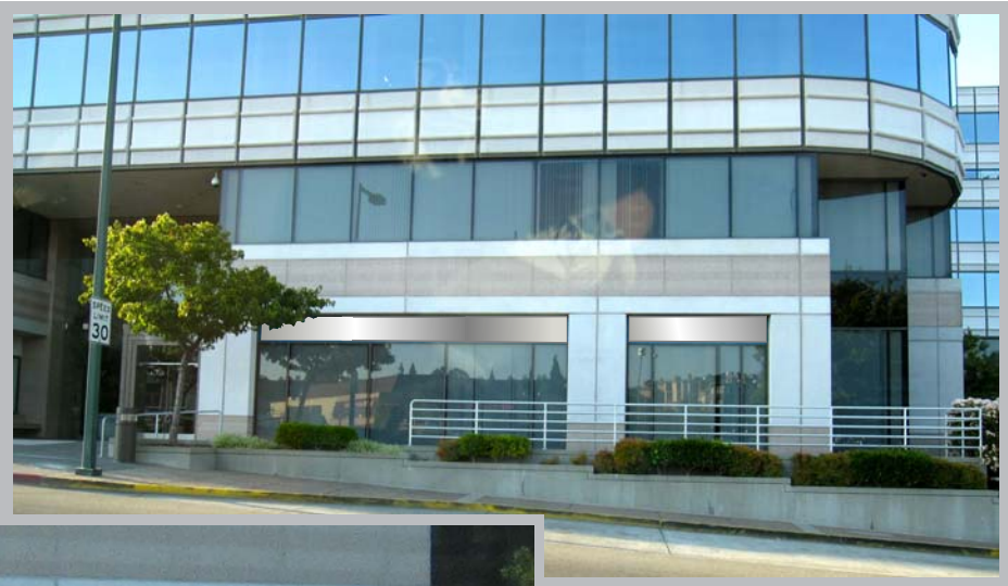
1331 | MT. DIABLO VIEW | EAST END OF BUILDING
