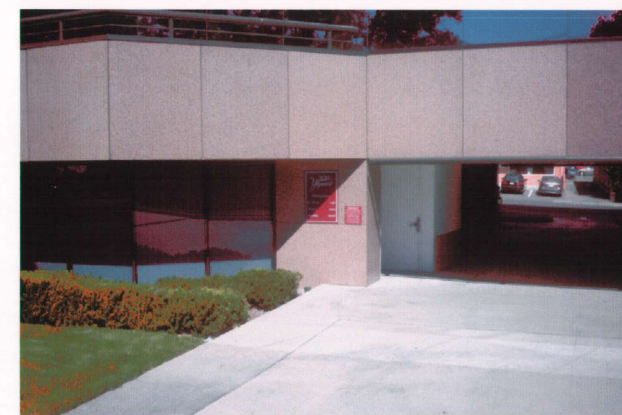
Existing sign @ P1b's location
