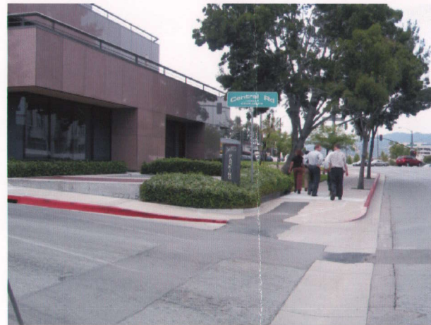
P3: Existing sign
