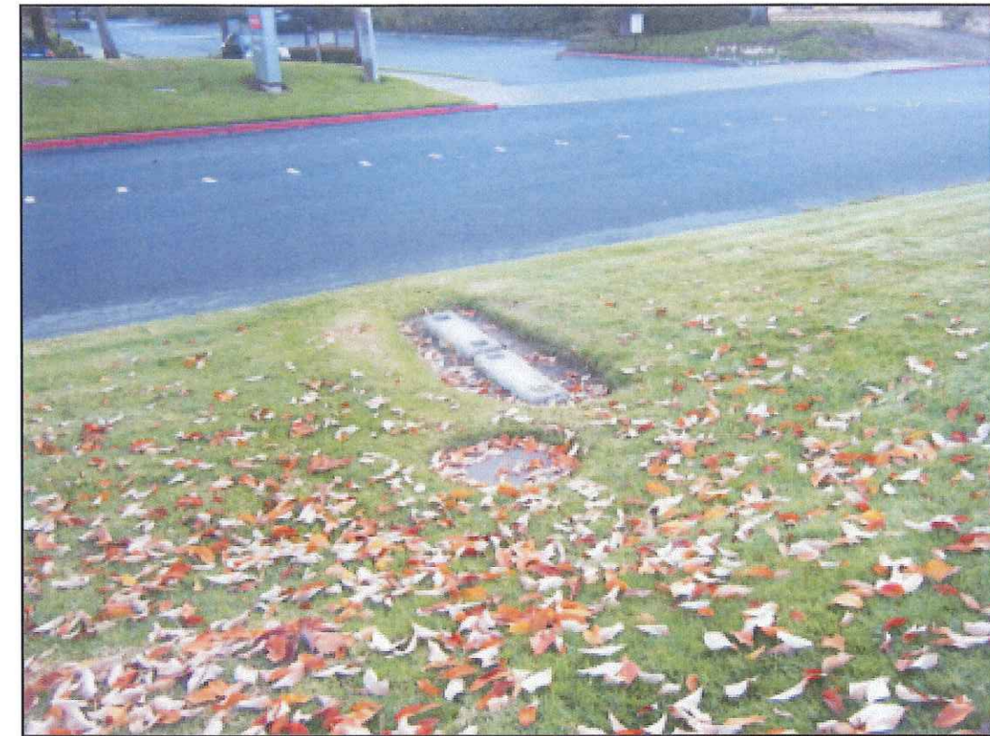
REPAIR EXISTING LANDSCAPE
