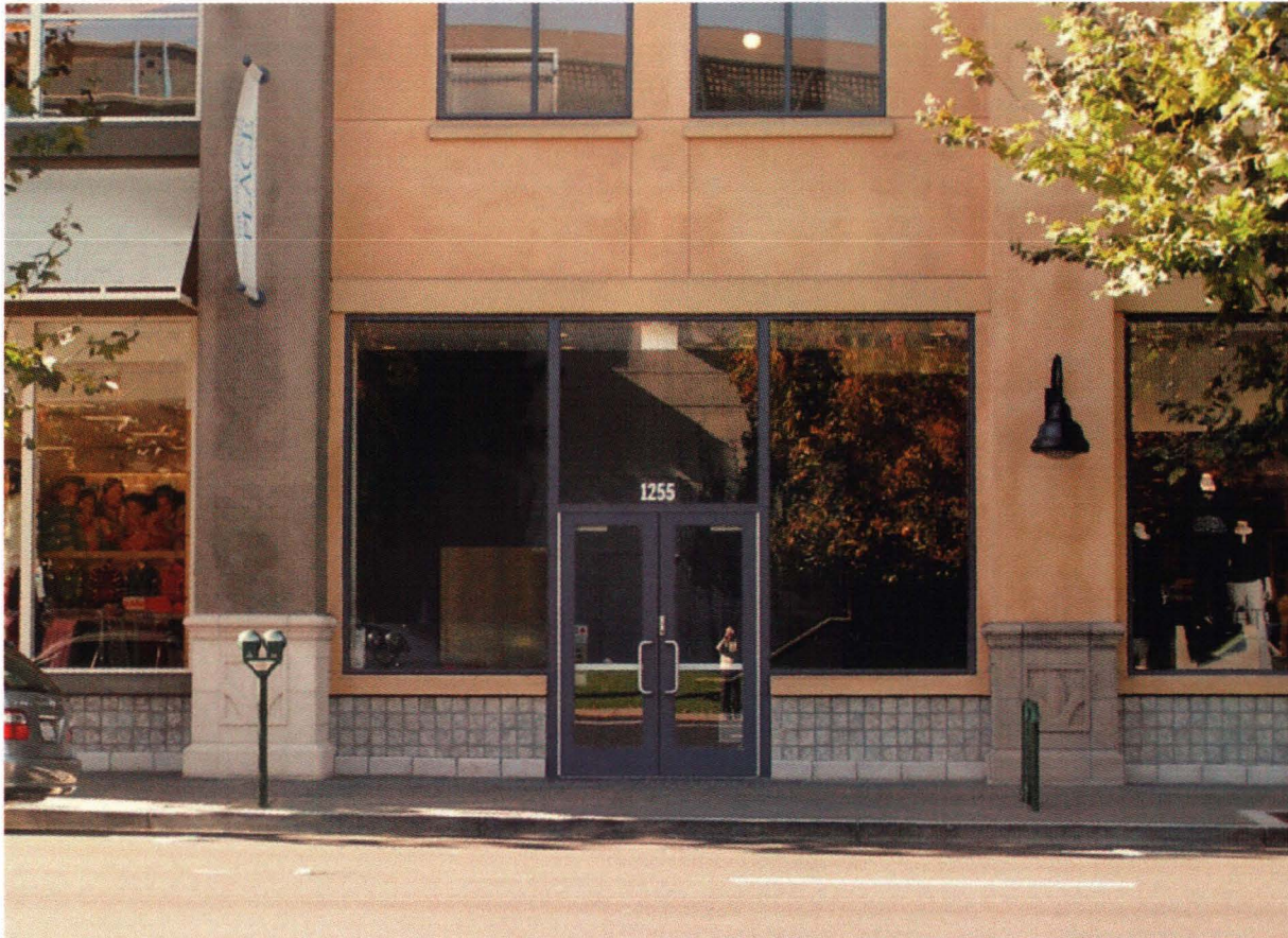
1255 S. MAIN ST. - 2nd FLOOR TENANT ENTRANCE
