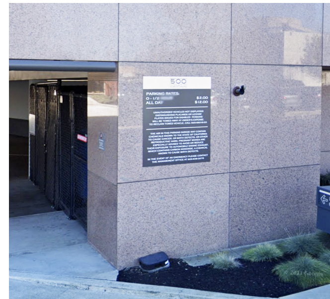
R1 Existing Photo
