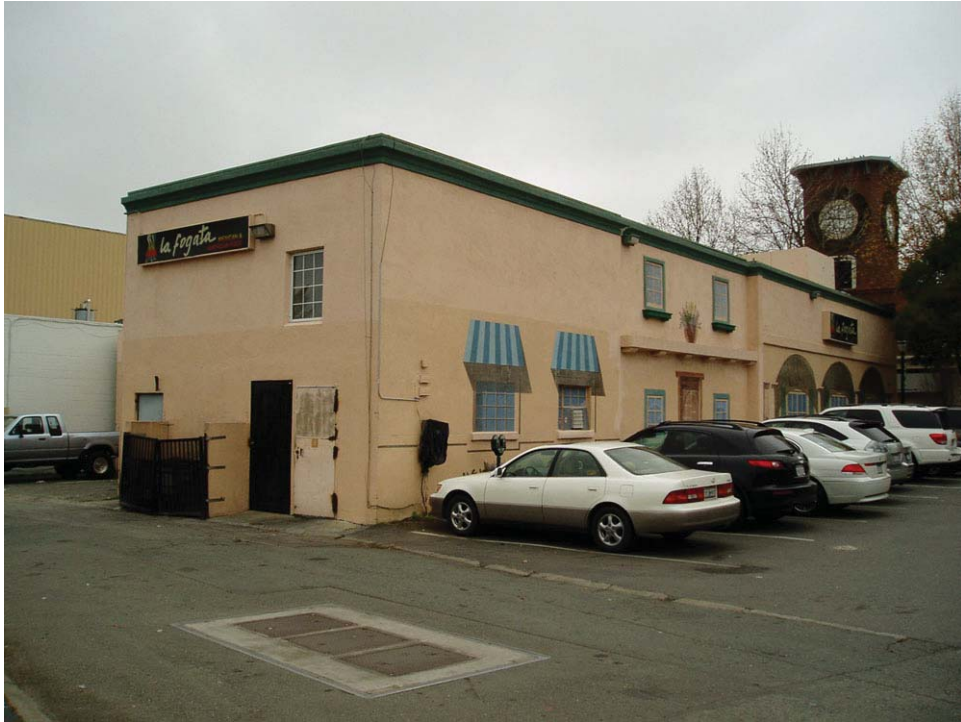
La Fogata Restaurant, Rear View
