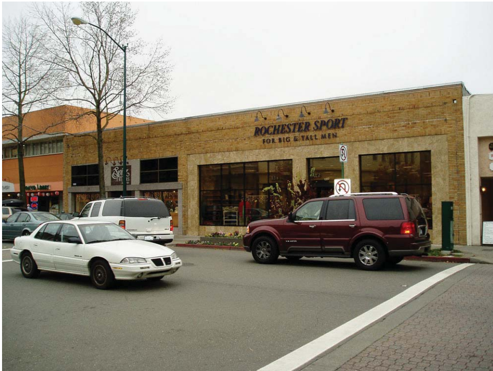
Westerly View from N. Main Street
