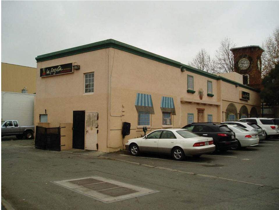
La Fogata Restaurant, Rear View
