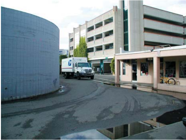
Truck access along Commercial Lane
