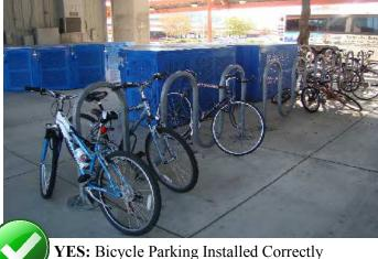
**YES:** Bicycle Parking Installed Correctly (Enough room to store bikes and access lockers)
