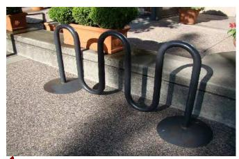
NO: Bicycle Rack Not Installed Correctly (No room between rack and wall to store a bike)
