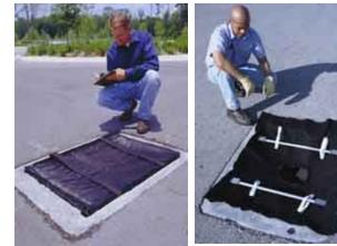
To protect <u>curb inlets without grates</u> where water flow is critical, use the following inlet protection. It is designed with a 3-dimensional high flow outer layer which encloses a multi-dimensional inner layer allowing high flow volumes to continue through the filter.
